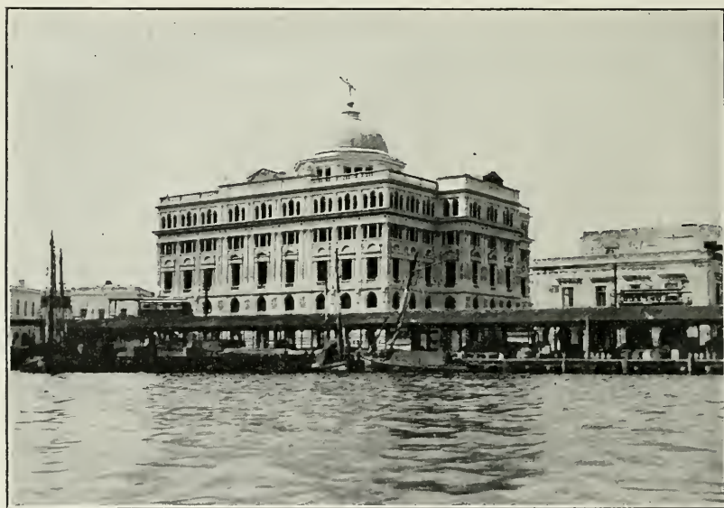
THE NEW PRODUCE EXCHANGE BUILDING IN THE CITY OF HAVANA—IT COST $600,000 GOLD AND WAS OPENED IN MARCH, 1909.
